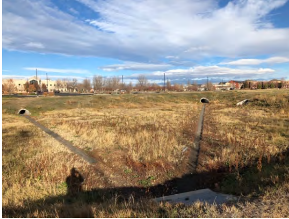
7. View of drainage basin and associated culverts and overflow riser, located along the southeastern portion of the site (facing north).
