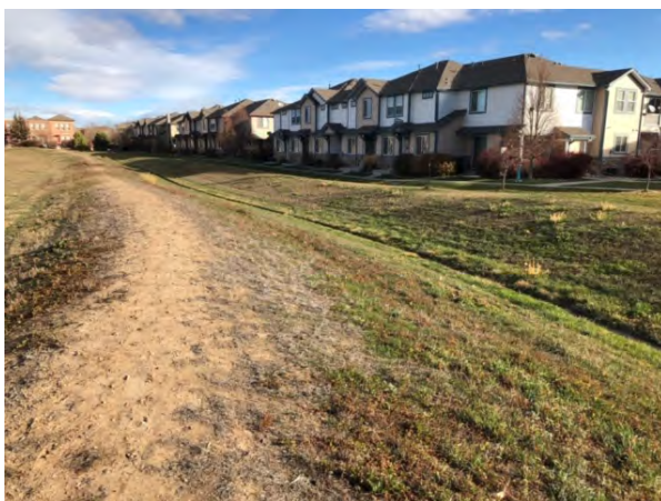
11. View of concrete lined drainage ditch located along the eastern boundary of the site (facing northeast).
