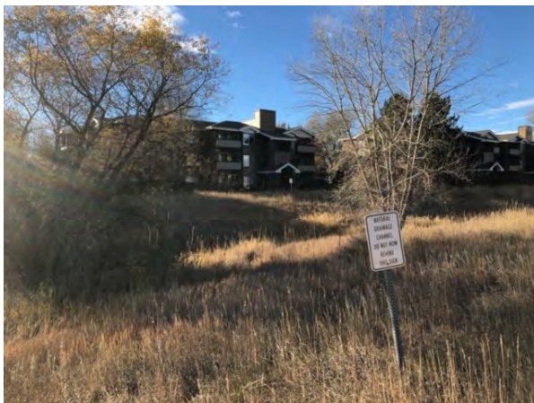
5. View of Foothills Channel to the adjacent south of the site, followed by multi-family residential property to the south (facing south).
