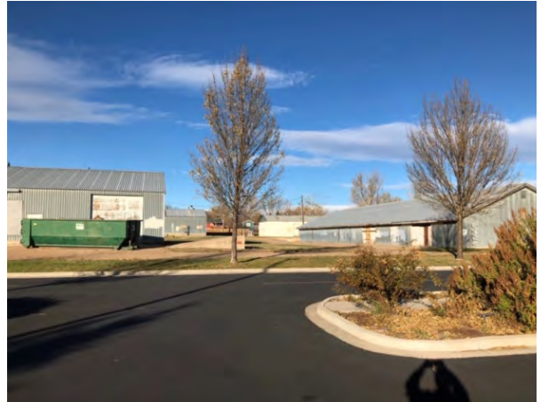
4. View of former CSU Agricultural Research Facility to the adjacent west of the site (facing west).
